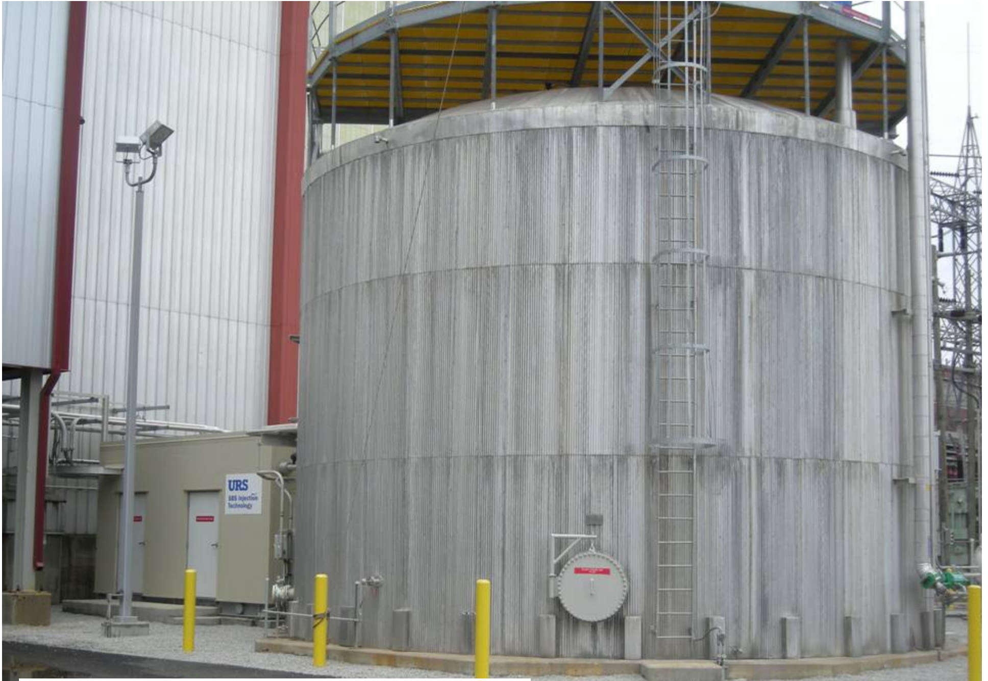
Solution Storage Tank and Injection Skid
